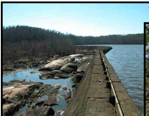
Great Falls Divergence Dam ...on an average day.
